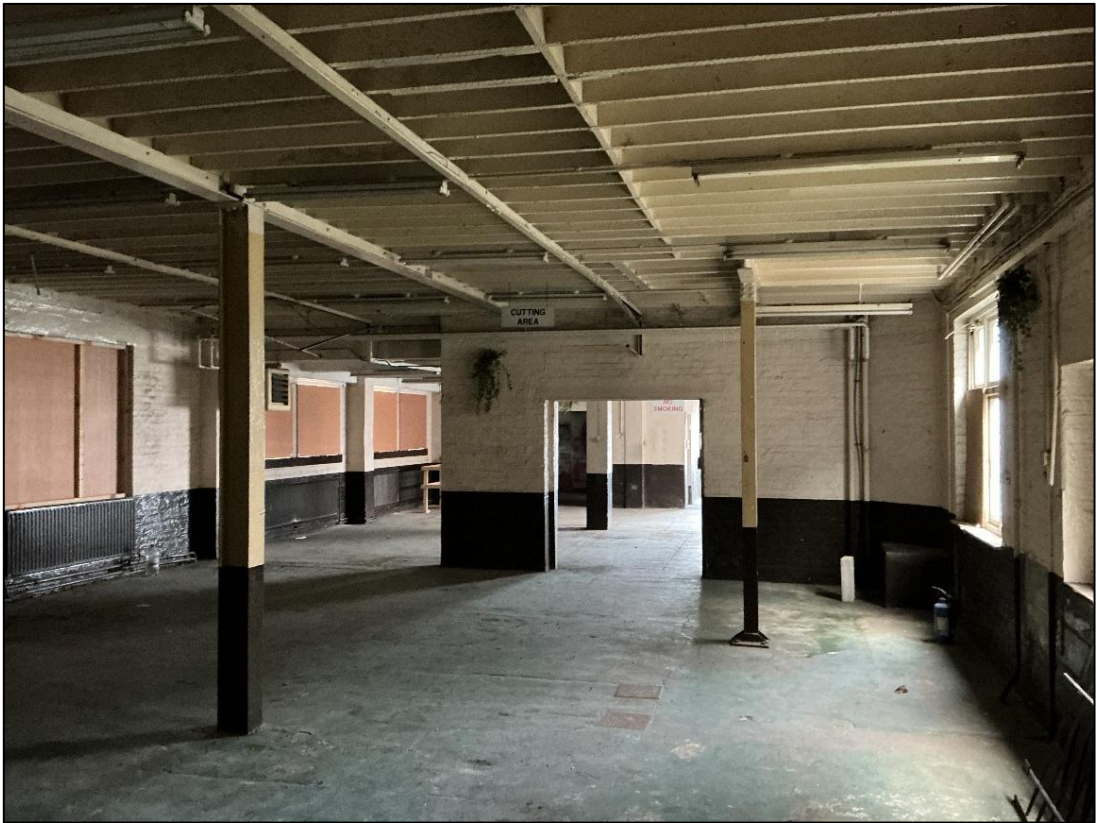
Figure 5: Existing Warehouse Ground Floor – General Internal Condition
