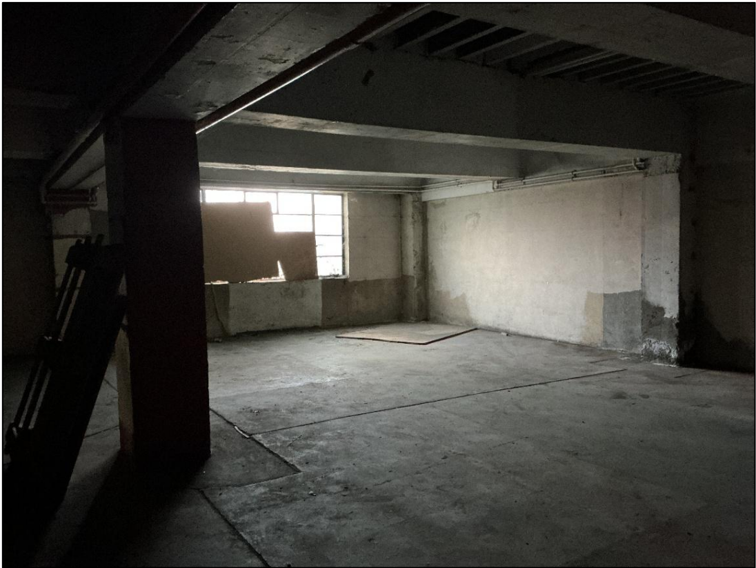
Figure 7: Existing Warehouse Basement – General Condition
