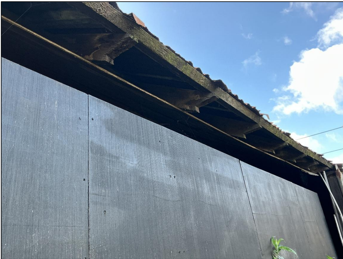
Figure 10: Roof Condition of Existing Steel Shed
