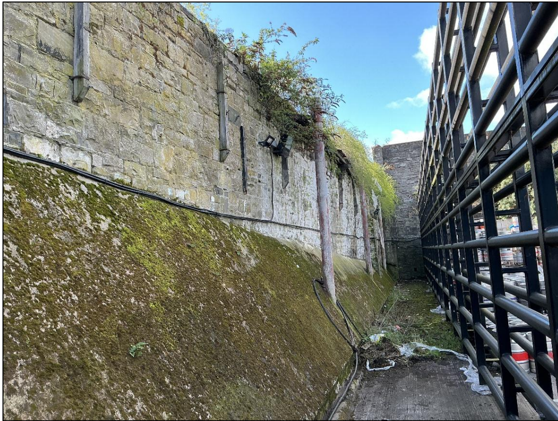
Figure 17: Existing Retaining Wall – Northern Boundary
