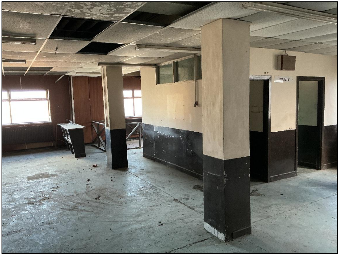
Figure 8: Existing Warehouse Upper Floor – General Condition
