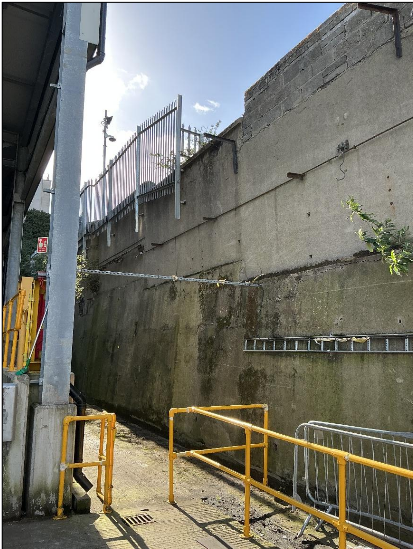
Figure 15: Existing Retaining Wall – Eastern Boundary
