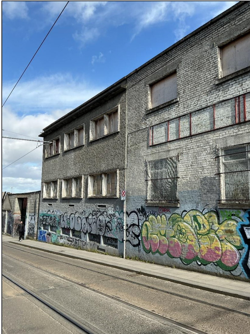
Figure 20: Western External Façade of Existing Building and Boundary Wall to Steevens Lane
