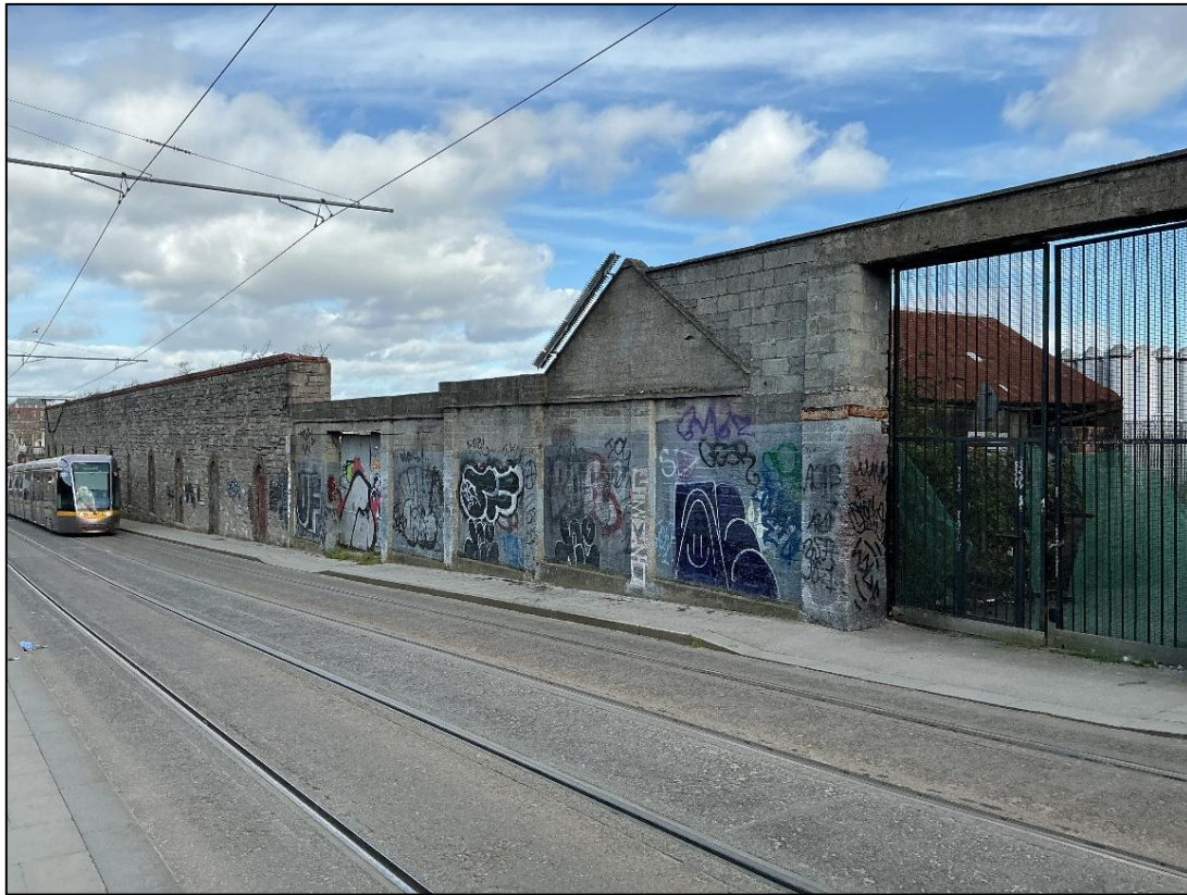
Figure 21: Boundary Wall to Steevens Lane – looking east
