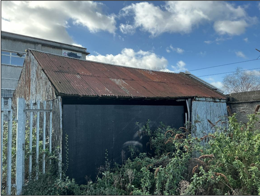
Figure 9: South External Façade of Existing Steel Shed
