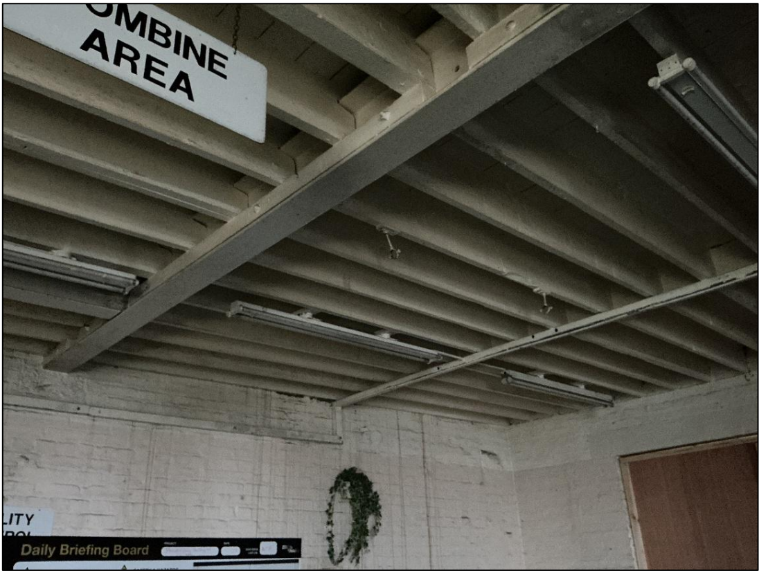
Figure 6: Existing Warehouse Ground Floor Interior Ceiling Framing
