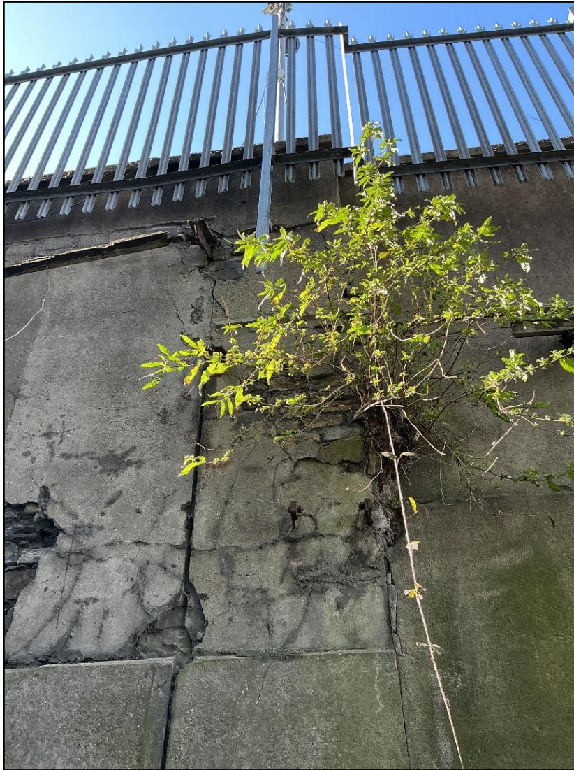
Figure 16: Existing Retaining Wall – Eastern Boundary (zoomed in structural condition)
