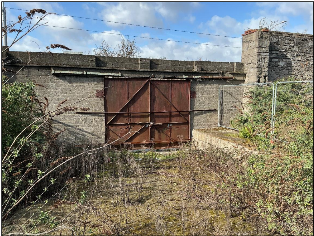
Figure 11: Northernmost Access Point to Steevens Lane – Looking West
