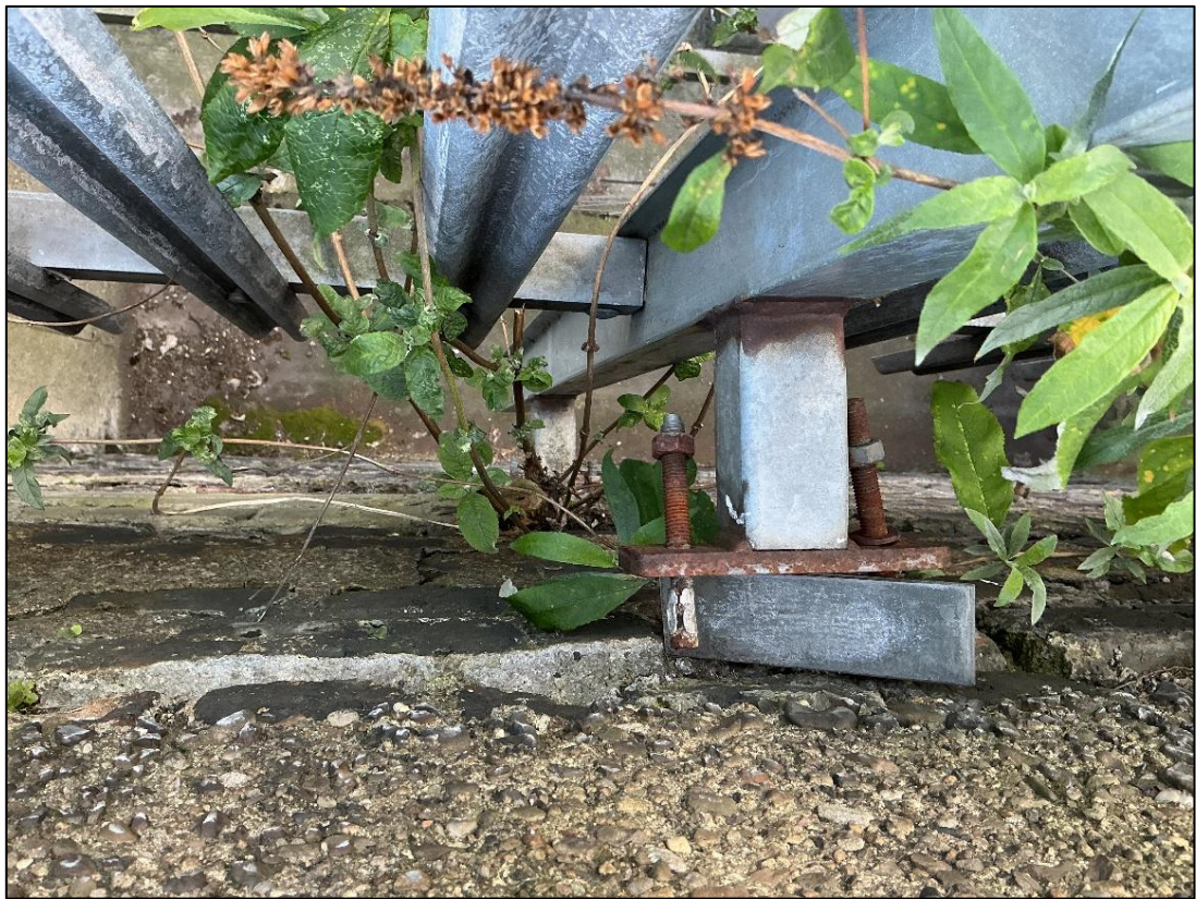
Figure 13: Steevens Lane Main Gate Structural Condition
